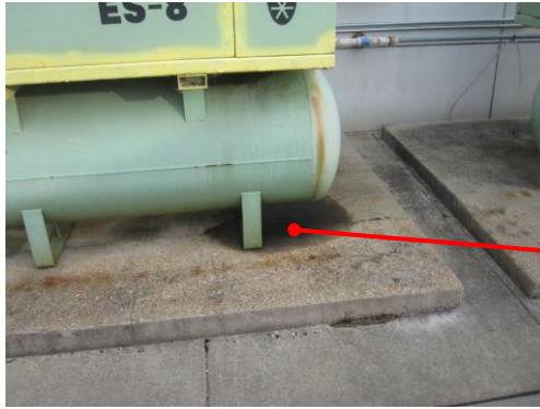
Oil leaking from outdoor compressor
