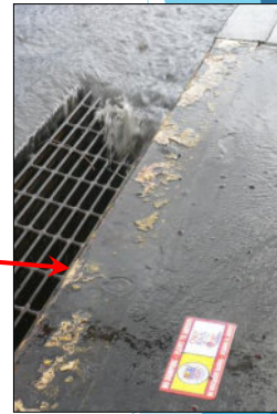
Storm sewer inlet
